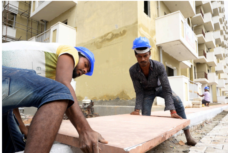
Covering up the storm drain
