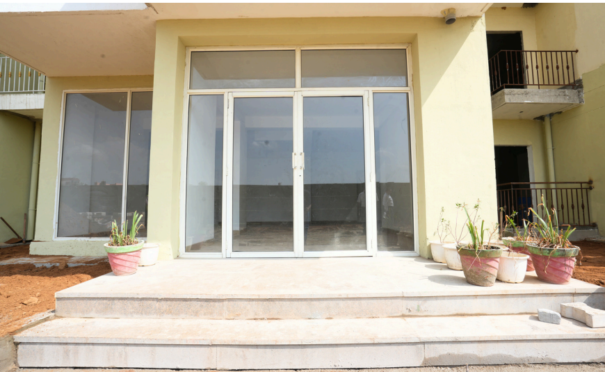
Entry of Tower S
