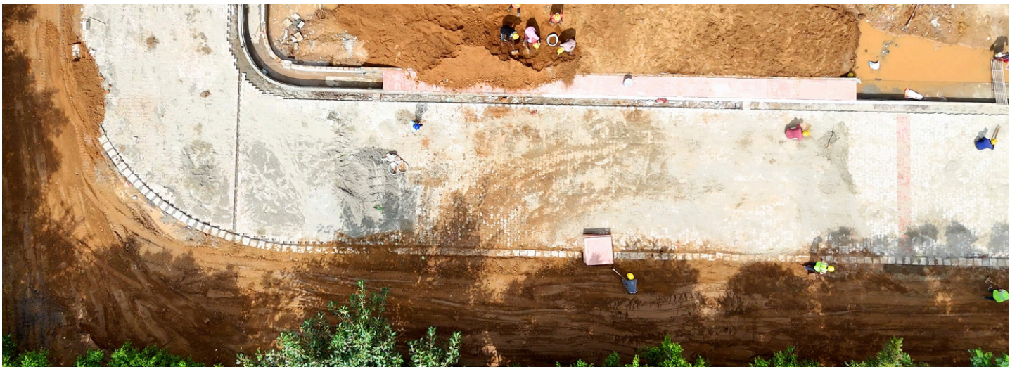
Top view showing the road, drain, green area and the boundary
