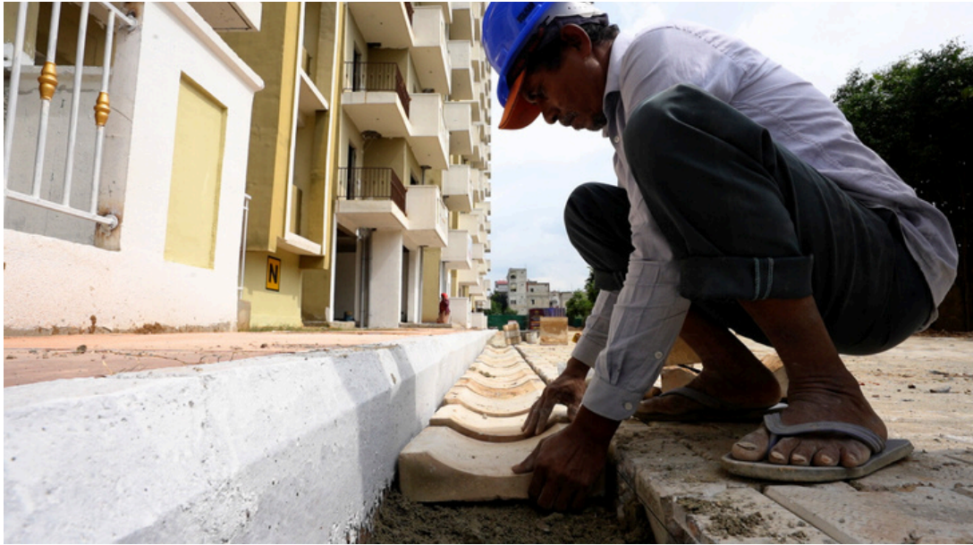
finishing the road work with saucer drain
