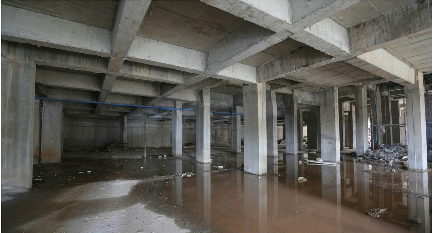
basement 1 car parking area
