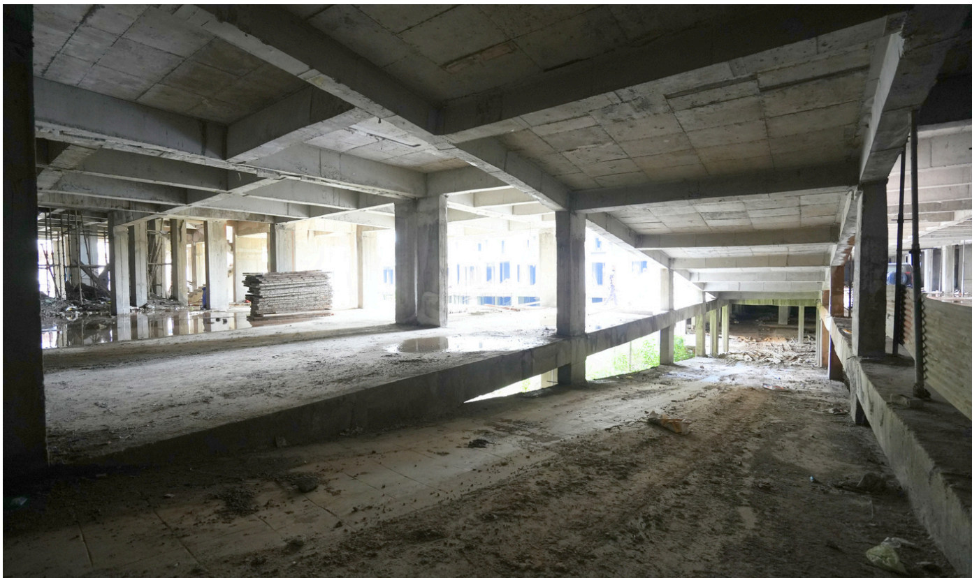
ramp from basement 1 to basement 2
