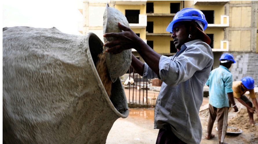
mixing cement & sand for plaster work
