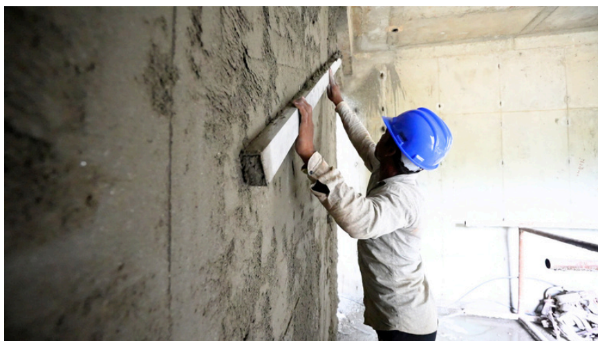
plaster work inside the apartment
